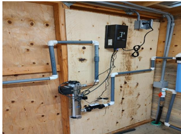
Water Filtration System Located inside Pumphouse. Plumbing of Viqua Pro 10 UV light system inside Pumphouse.
