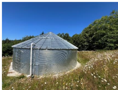
Corrugated steel tank with bladder liner
