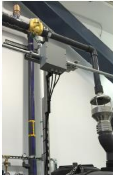
FIGURE 6: SOLENOID VALVE AND AIR GAP
