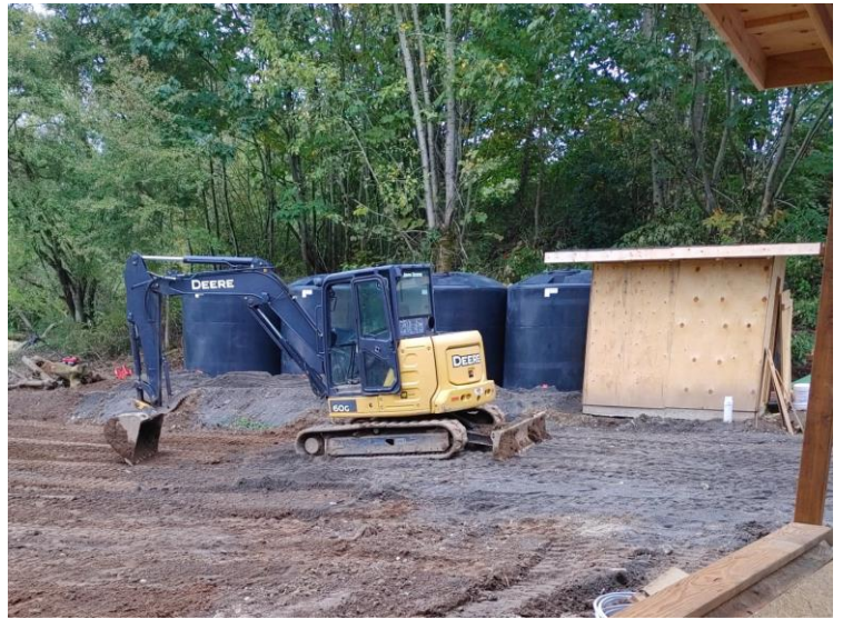
Site construction of RWH system with pumphouse.
