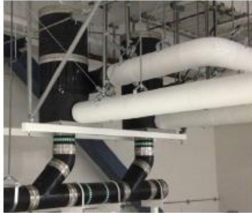
FIGURE 2: WISY WFF300 VORTEX FILTERS
