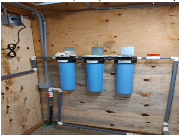
Water Filtration System Located inside Pumphouse. Plumbing of Viqua Pro 10 UV light system inside Pumphouse.
