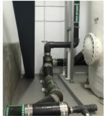
FIGURE 5: DUPLEX BOOSTER PUMP SKID
