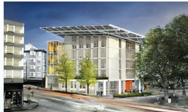
Bullitt Center, Seattle, WA. The greenest commercial building in the world, with a 56,000-gallon cistern designed for potable use. www.bullittcenter.org; credit Miller Hull Partnership.
