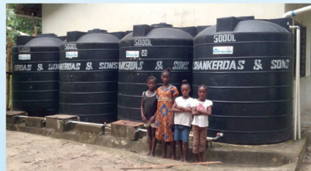
School, Makali, Sierra Leone. 20,000-liter rainwater storage for 90-inch annual rainfall. www.RainBank.info; submitted by Ken Blair.
