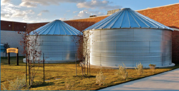
Carpenter Hill Elementary School, Buda, TX. 106,000 gallons of rainwater storage; photo by HarveyJack, wh 2 o.
