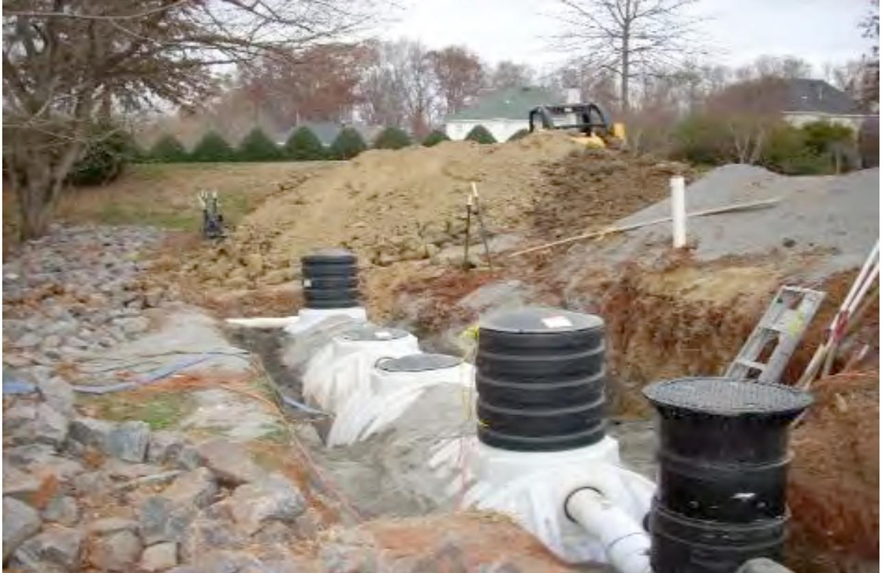
Figure 4.13 Below ground polypropylene tanks
