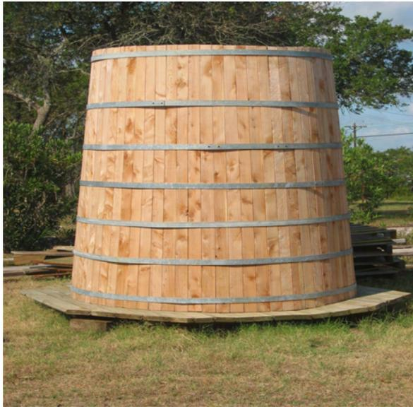
**Figure 4.15** Wooden aboveground tank
