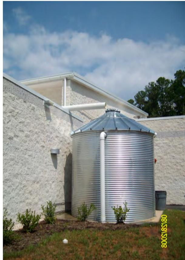
**Figure 4-14 Corrugated steel tank**
