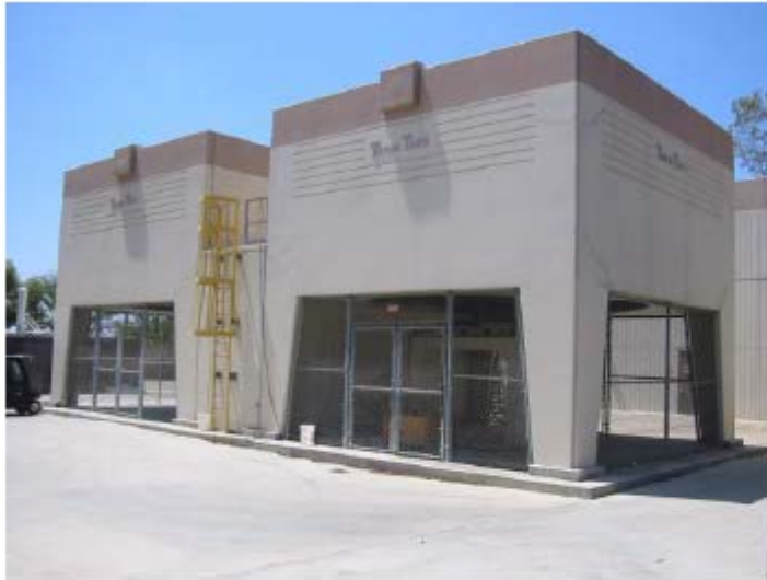
Concrete Tower Basin
